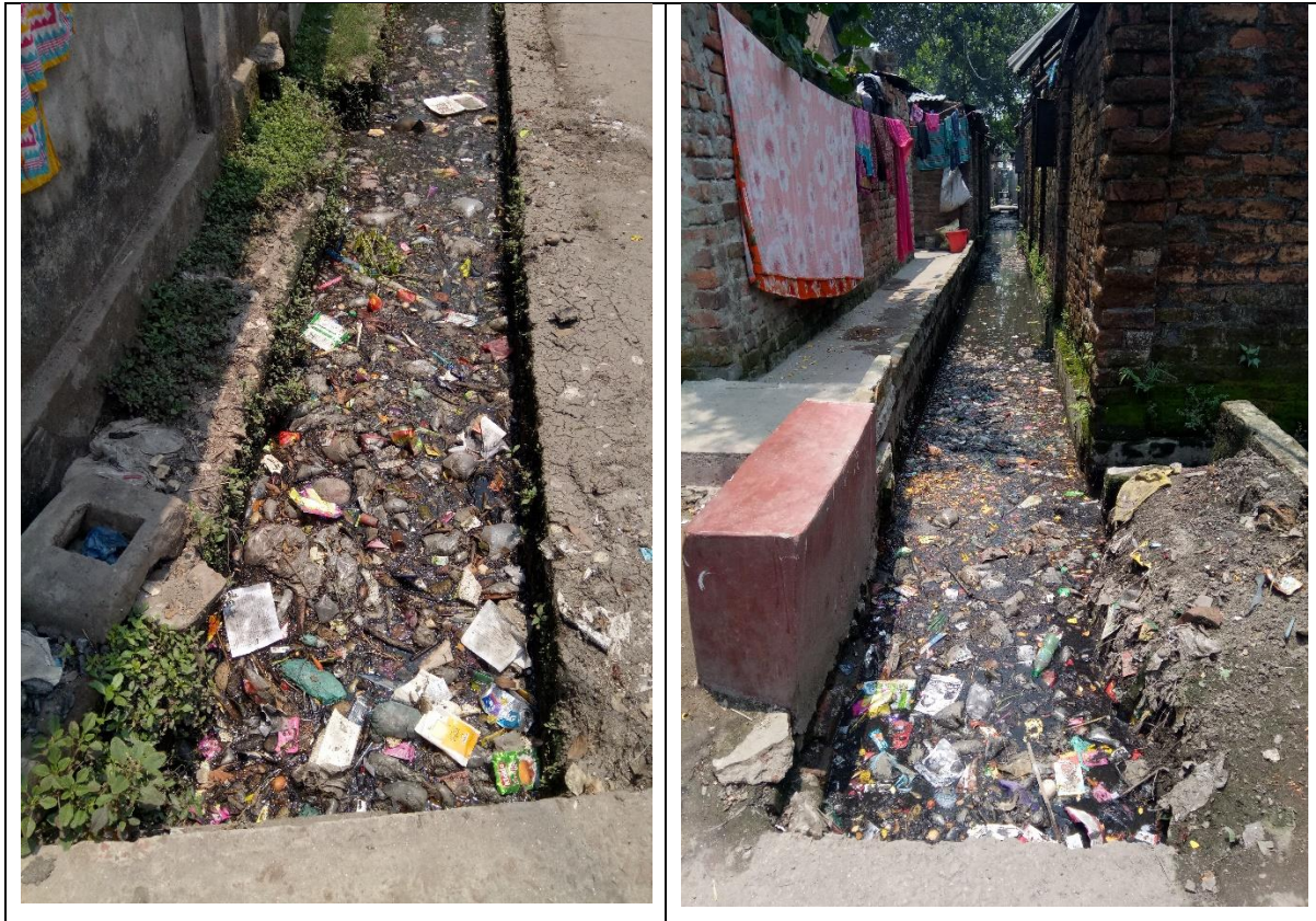
Figure 10.2: Dumping household solid waste directly to the drain (Saidpur Bihari camp)
